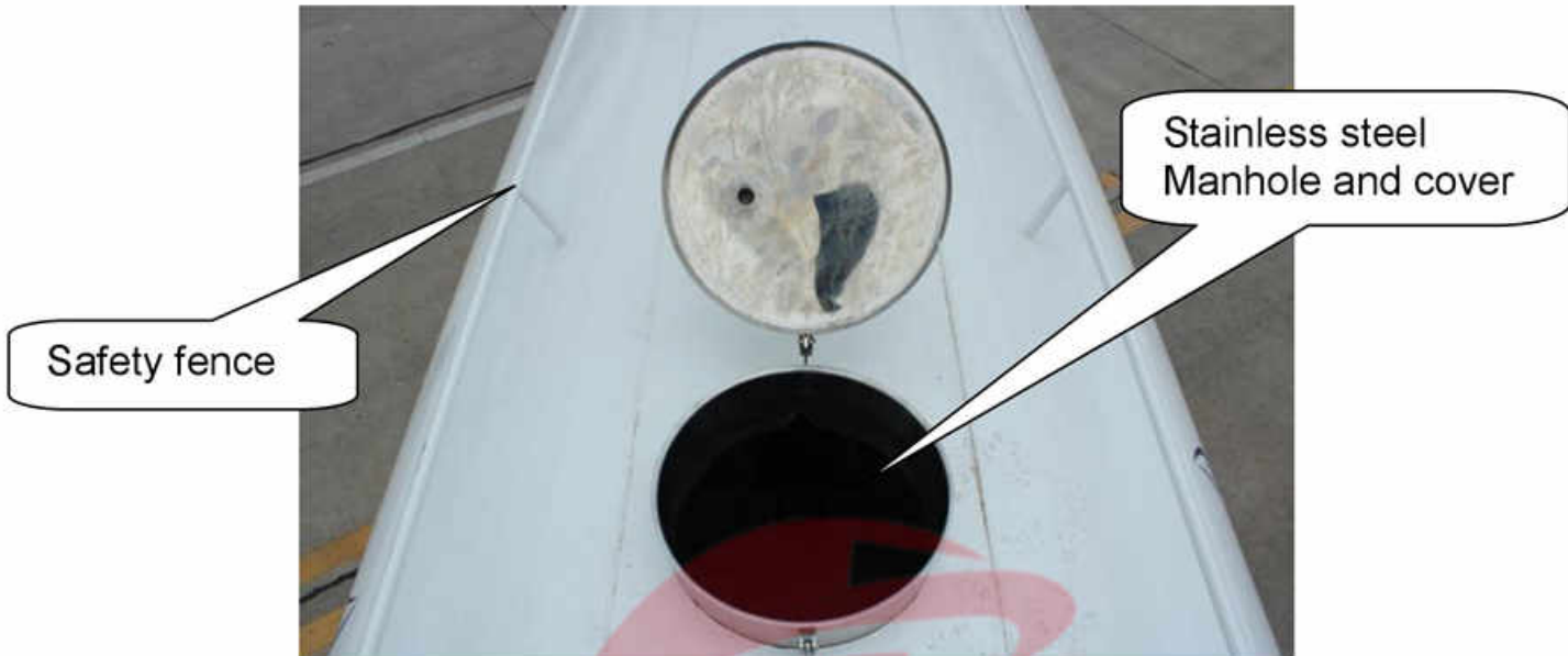
Top of the Tank: Stainless steel manhole and safety fence
